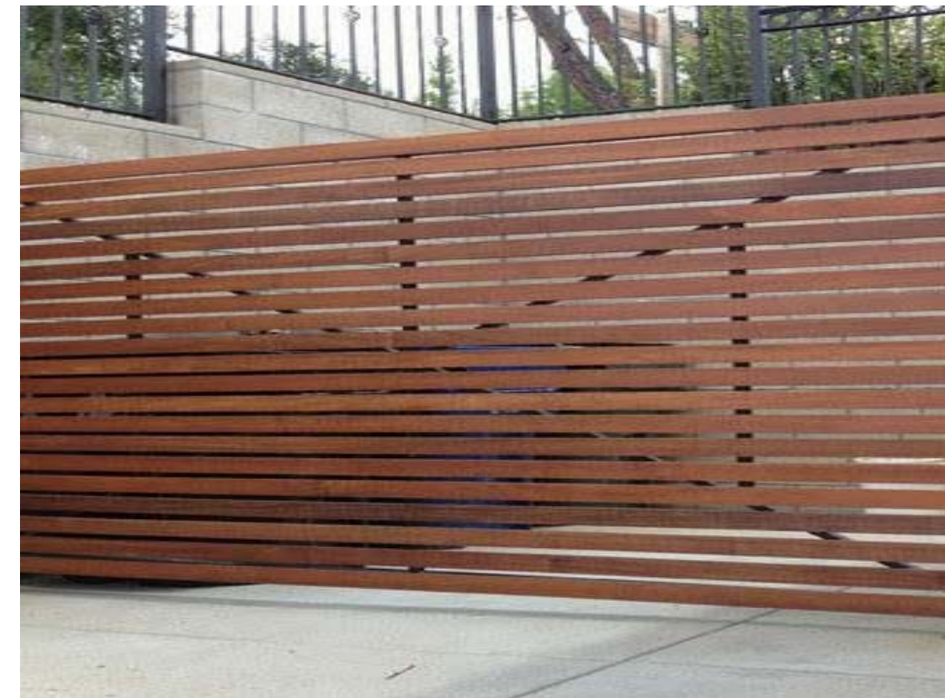
CEDAR FENCE ALONG PROPERTY LINE
