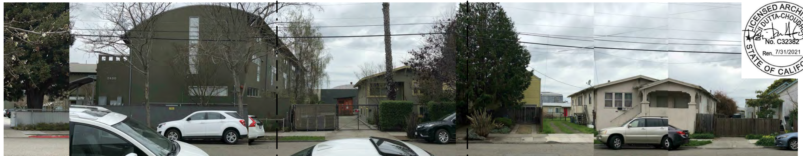
EXISTING WEST VIEW 2422 5TH STREET
