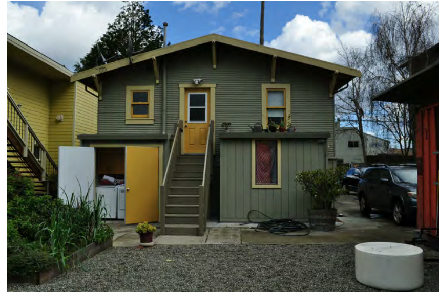
B - EXISTING BACK OF HOUSE
