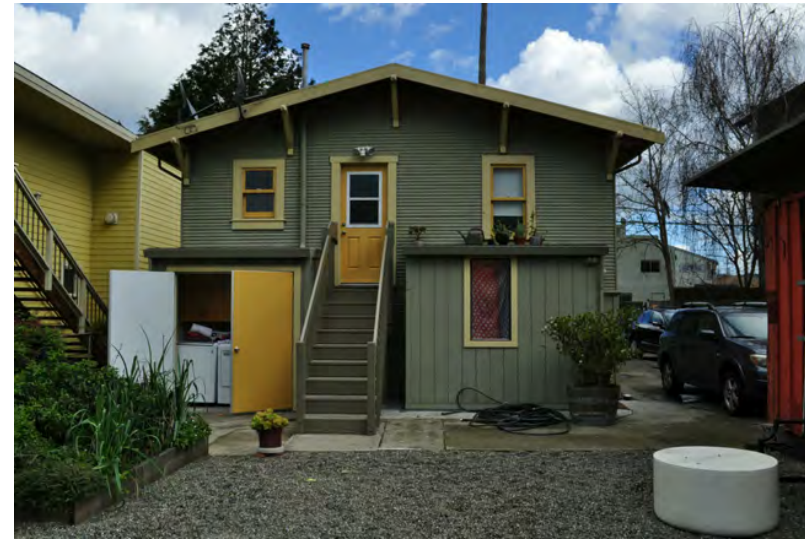
B - EXISTING BACK OF HOUSE
