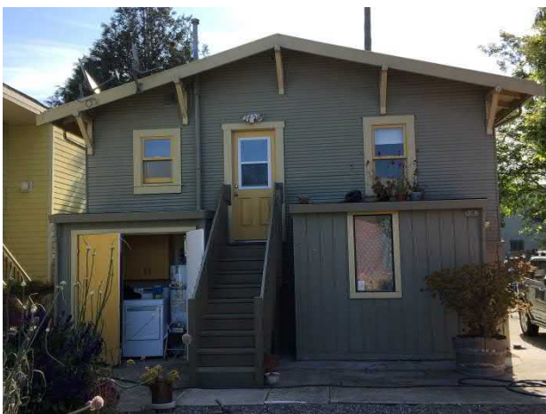
3. View of the subject property building (facing east)
