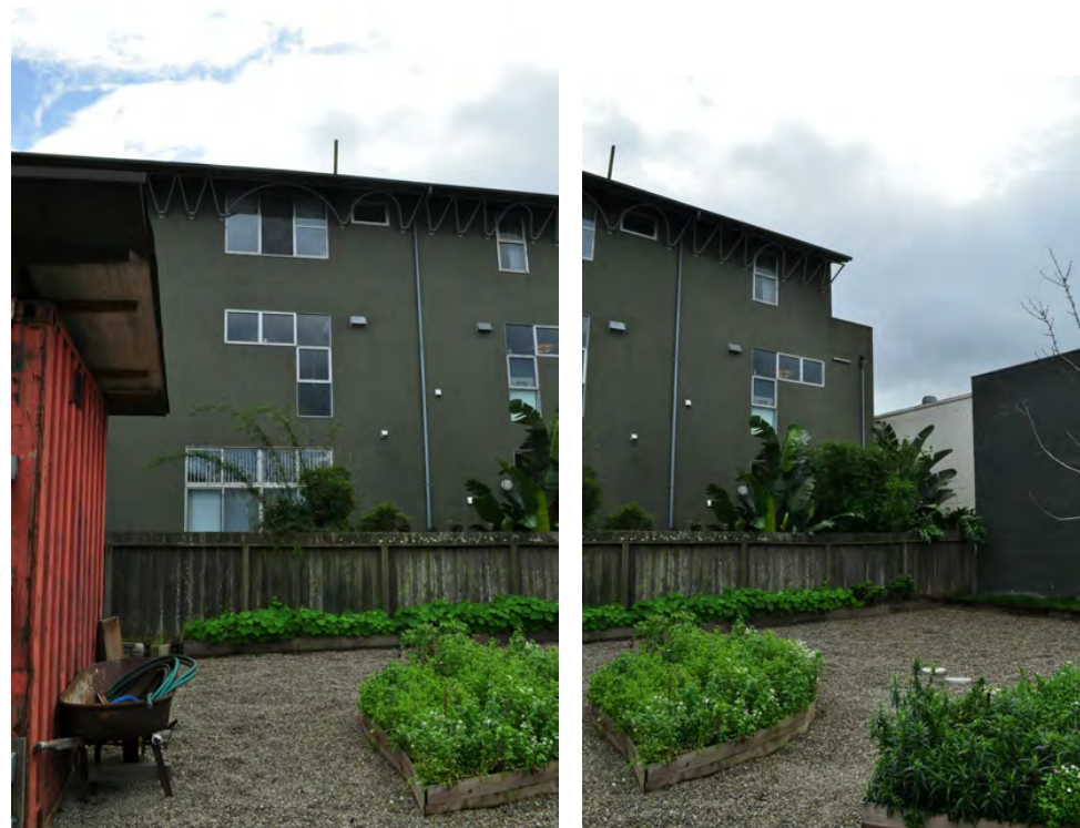
D,E - ADJACENT MULTI-FAMILY BUILDING
