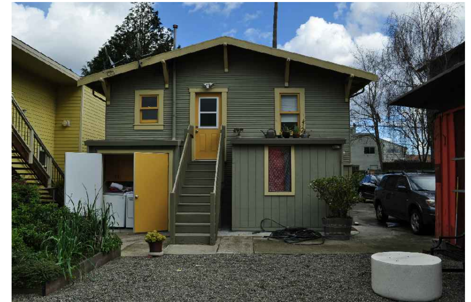
F - EXISTING BACK OF HOUSE
