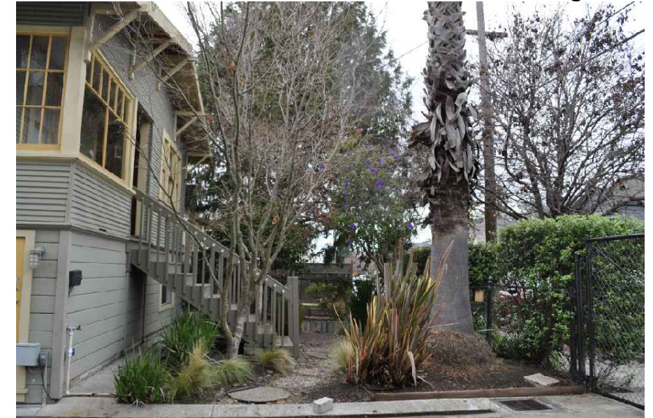
C - EXISTING FRONT YARD
