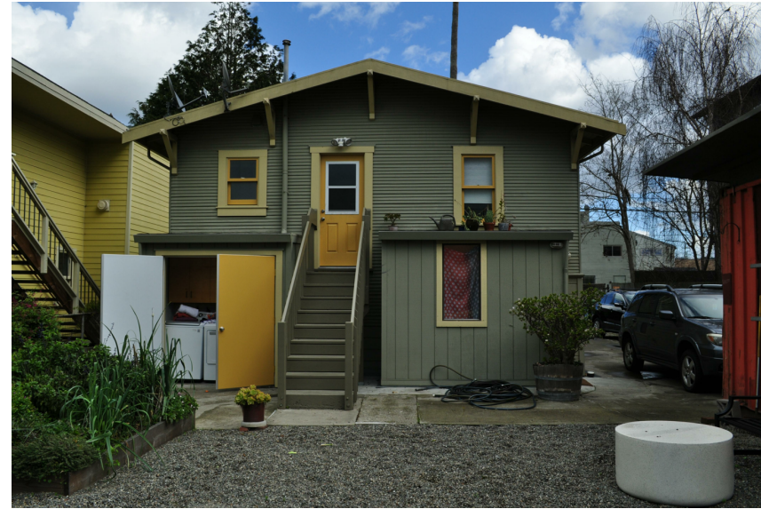
B - EXISTING BACK OF HOUSE
