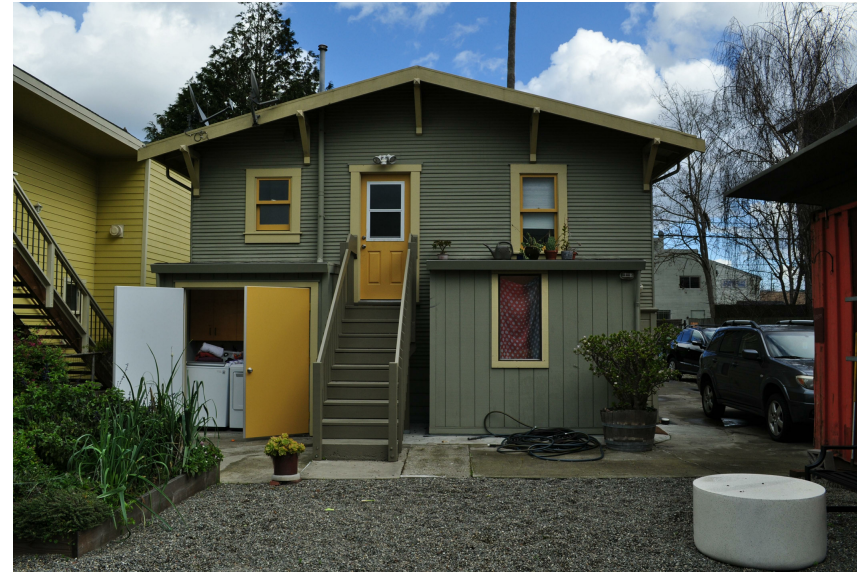
B - EXISTING BACK OF HOUSE
