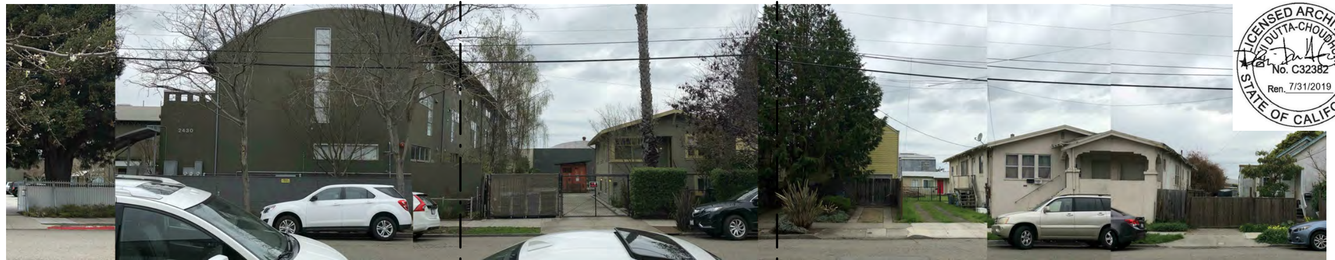
EXISTING WEST VIEW 2422 5TH STREET
