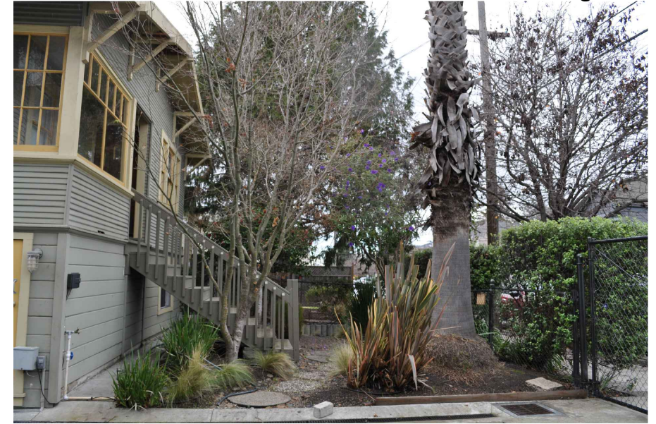
C - EXISTING FRONT YARD
