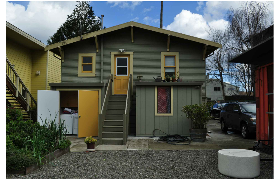
F - EXISTING BACK OF HOUSE
