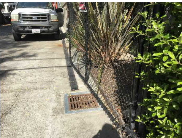
21. View of the stormwater drain
