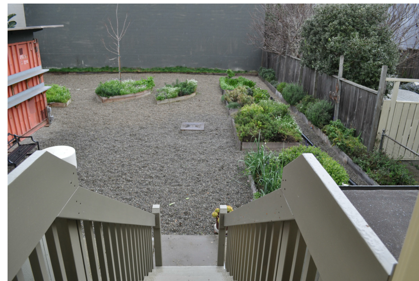
F - EXISTING REAR STAIR/YARD
