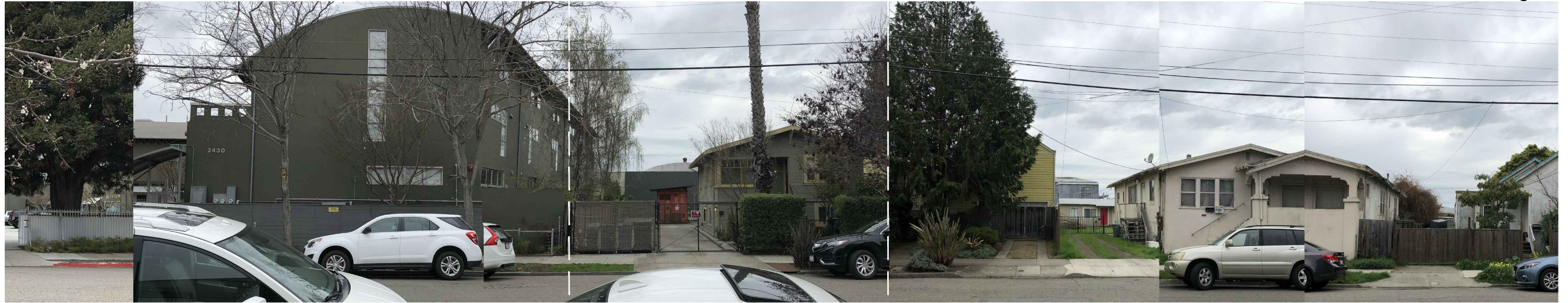
EXISTING WEST VIEW 2422 5TH STREET
