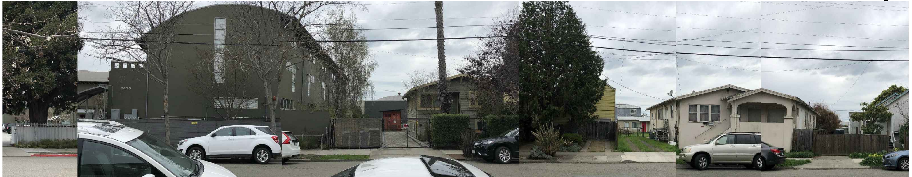
EXISTING WEST VIEW 2422 5TH STREET
