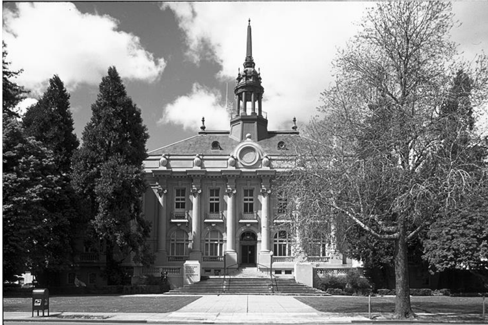
Berkeley's original City Hall is now a National Register-listed City Landmark and the site of the City Council's Tuesday evening meetings.
