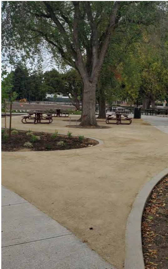
Decompose Granite (stabilized) pathways
