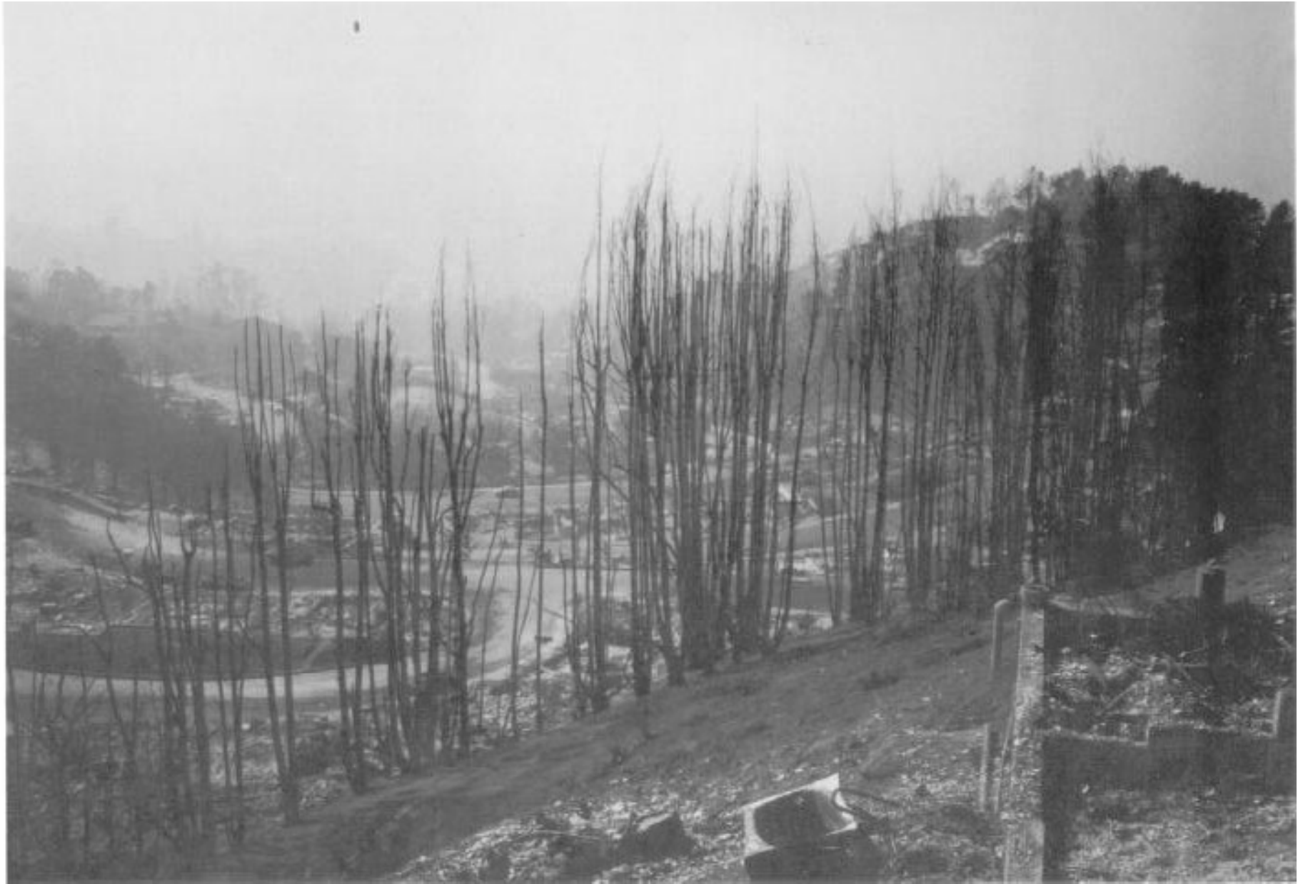
Total destruction of Hiller Highlands complex.
