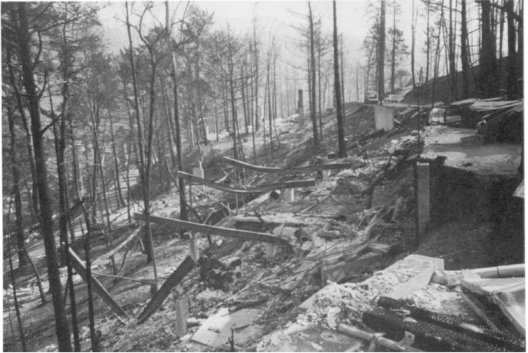
Buckled steel beams mark the location of a destroyed home on Buckingham Boulevard.
