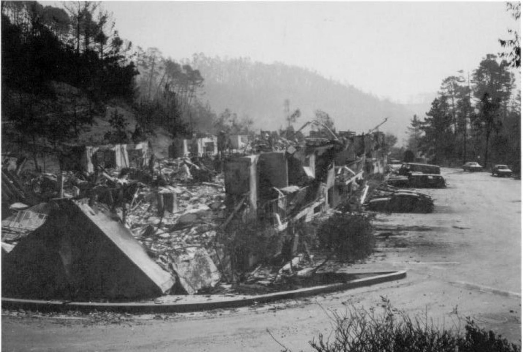
Ruins of the Parkwood Apartments; previously 4-story buildings.
