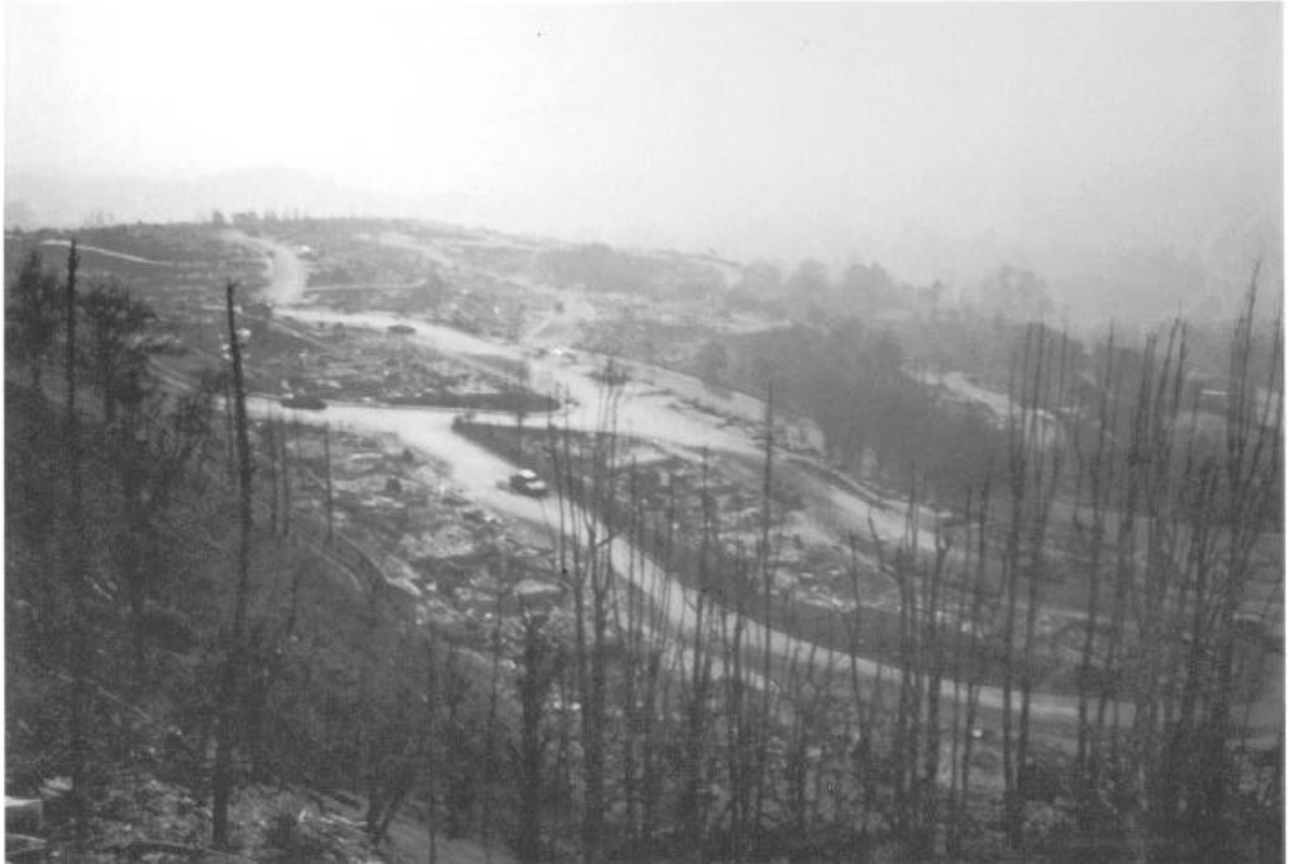
Total destruction of Hiller Highlands complex.
