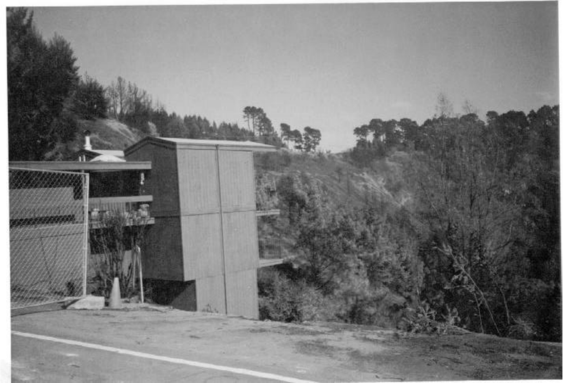
One of the few homes on Marlborough Terrace that was not destroyed by the fire. Houses on both sides burned to the ground.
