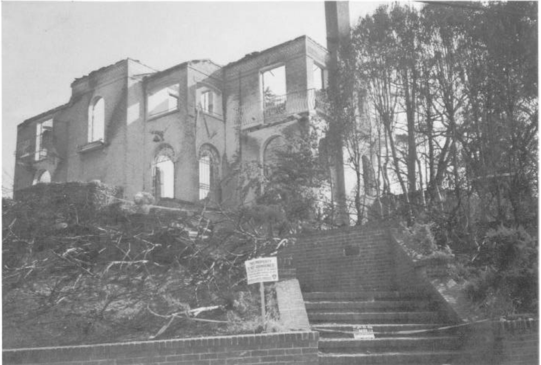
Ruins of large 2-story home in Rockridge district.
