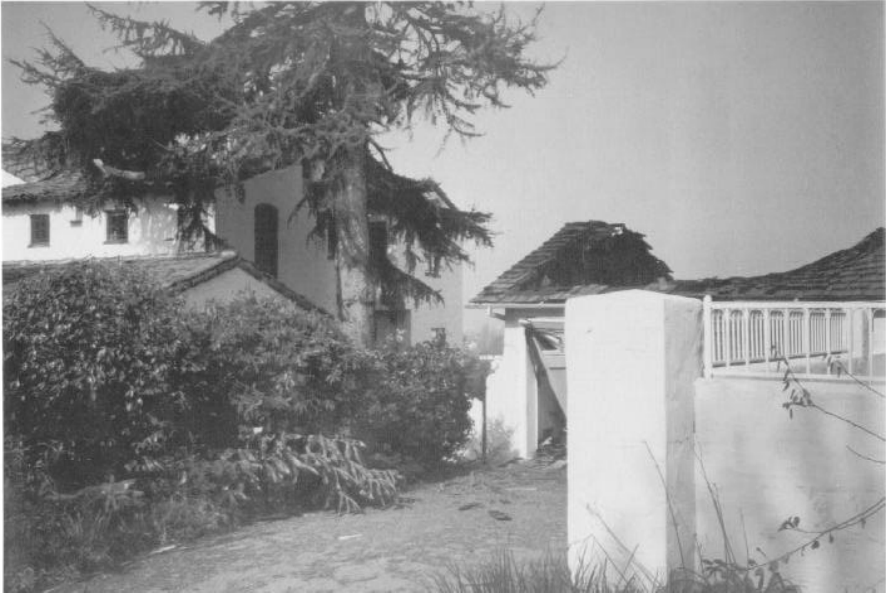
Home with wood shingle roof destroyed. Neighboring home with tile roof saved.
