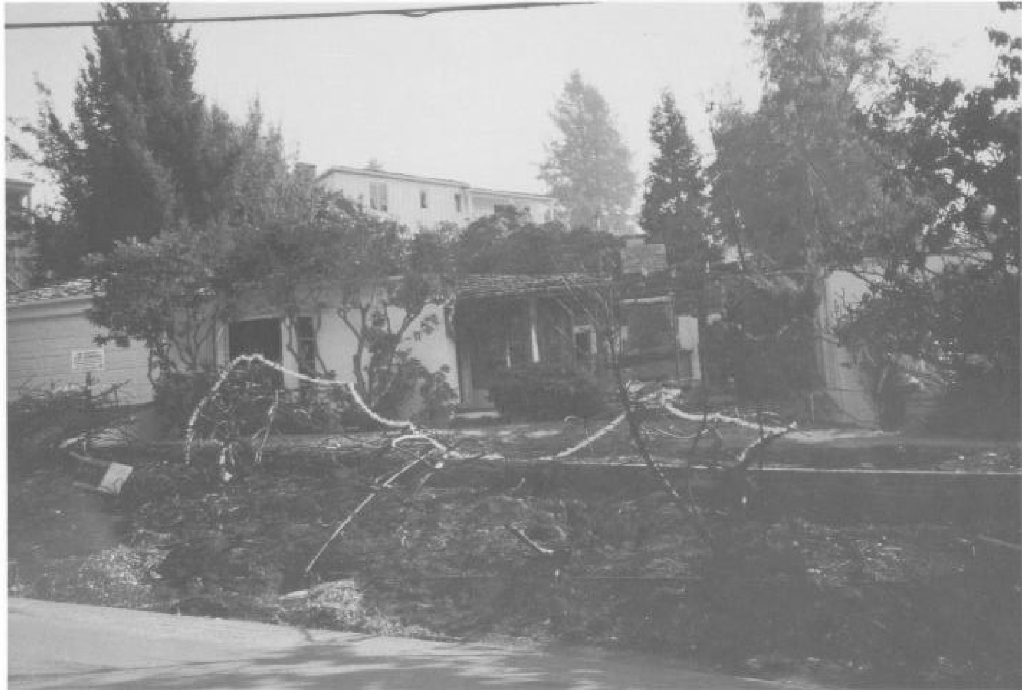
Home with wood roof burned off.
