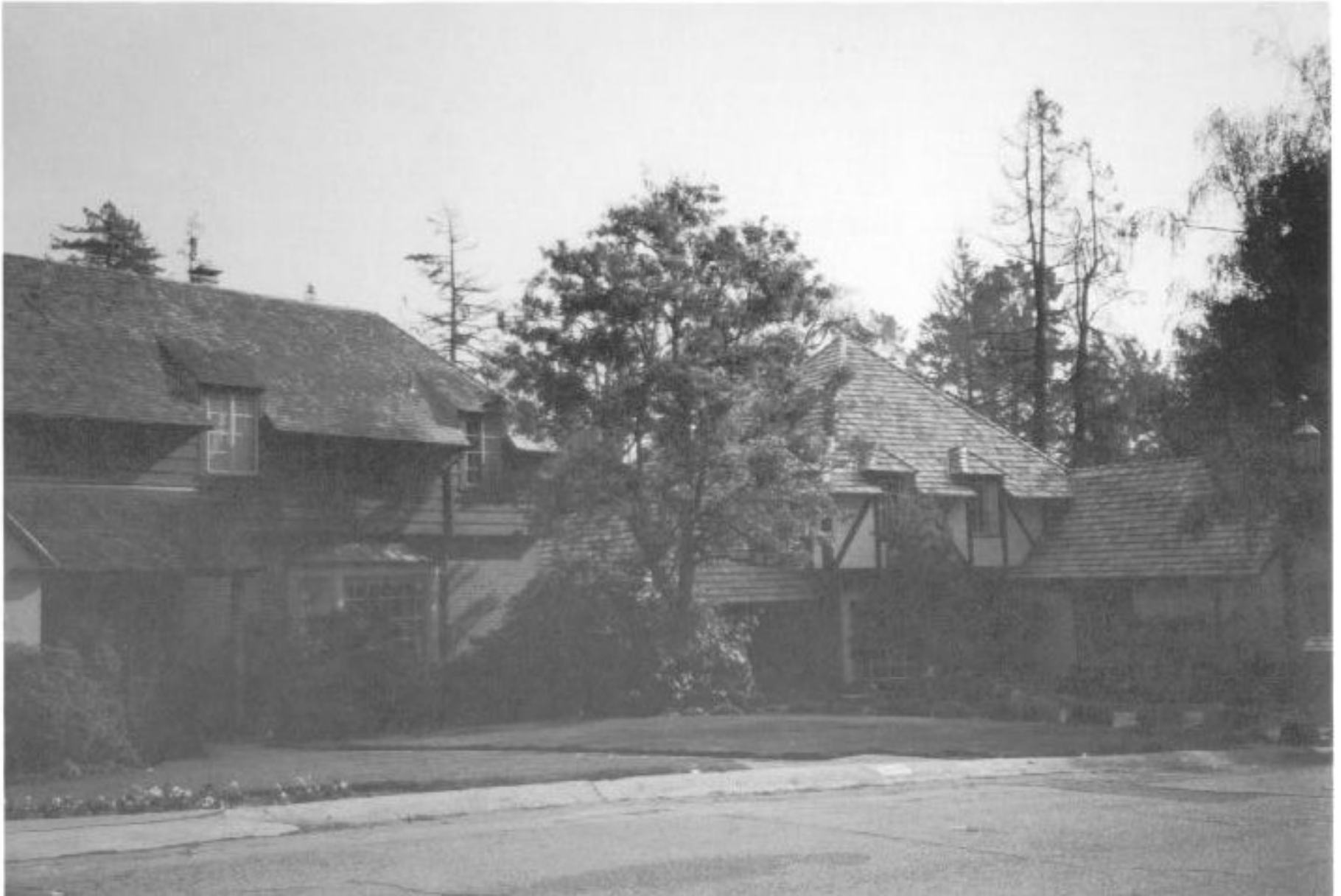
Examples of development in the fire area - wood shingle roofs.
