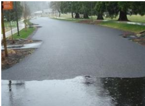
Figure 3-7, Porous Asphalt (adjacent to conventional asphalt)
