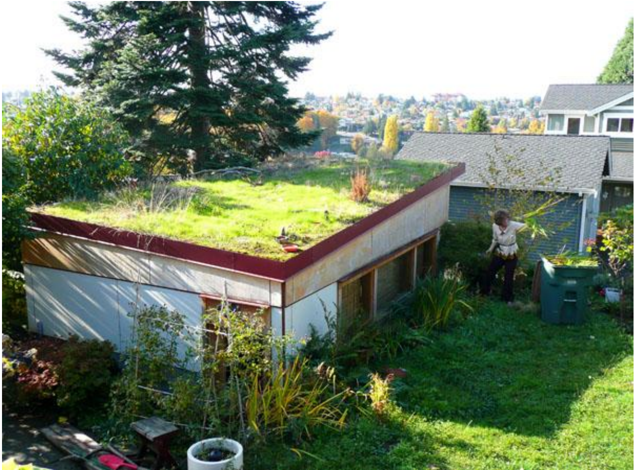
Figure 3-5, Garage Green Roof in Mount Baker
