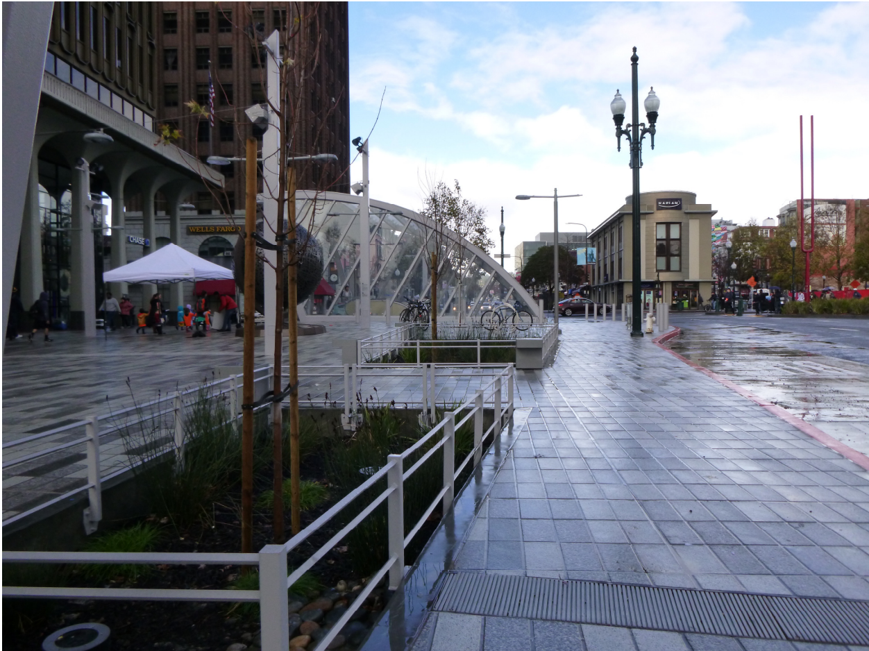
Figure 33 – Flow-through planters installed above the Downtown Berkeley BART Station treat runoff from Shattuck Avenue.
