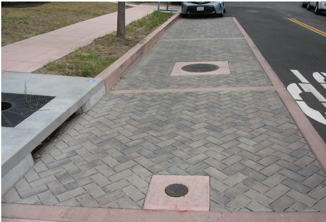
Figure 3 – The entire block of Allston Way between Milvia Street and Martin Luther King Jr. Way is paved with permeable pavers.
