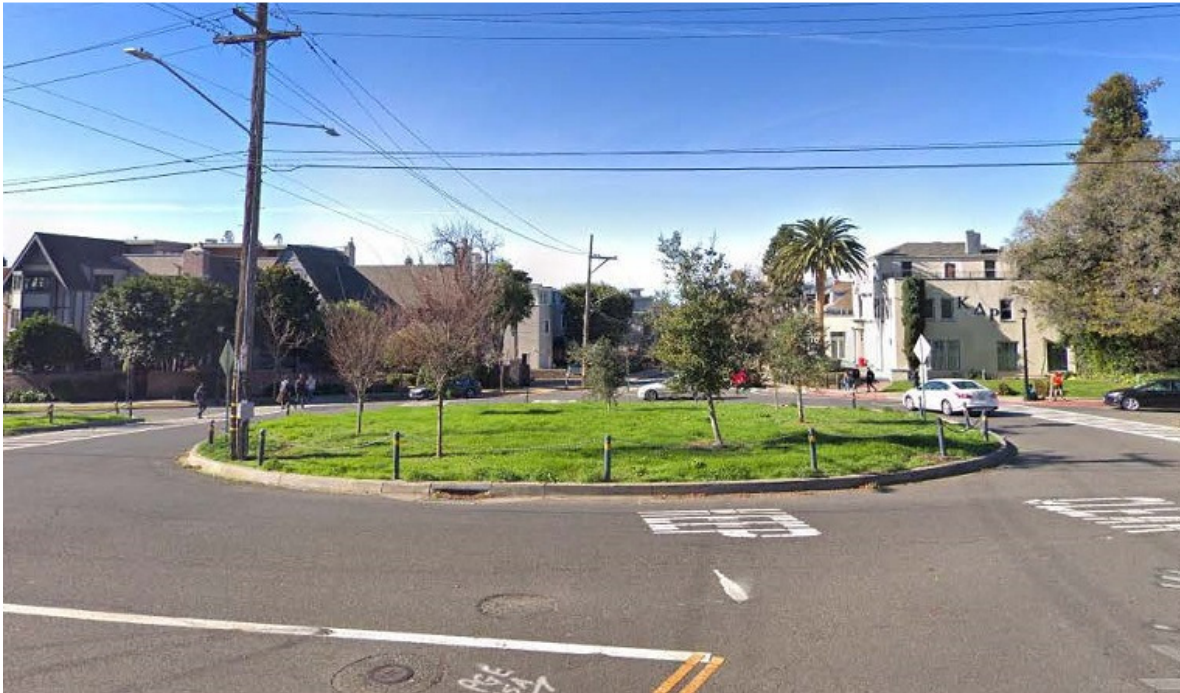
Figure 13 – The large grassy traffic circle at Piedmont Avenue and Channing Way could be retrofitted into a bioretention feature to treat runoff from the street.
