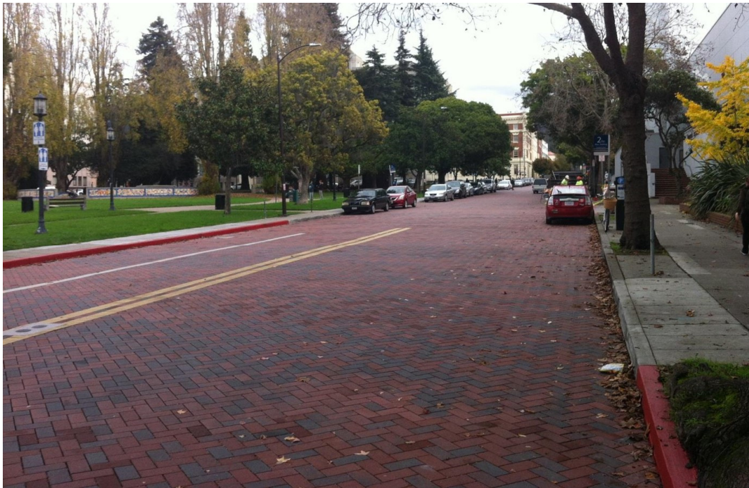
Figure 3 – The entire block of Allston Way between Milvia Street and Martin Luther King Jr. Way is paved with permeable pavers.
