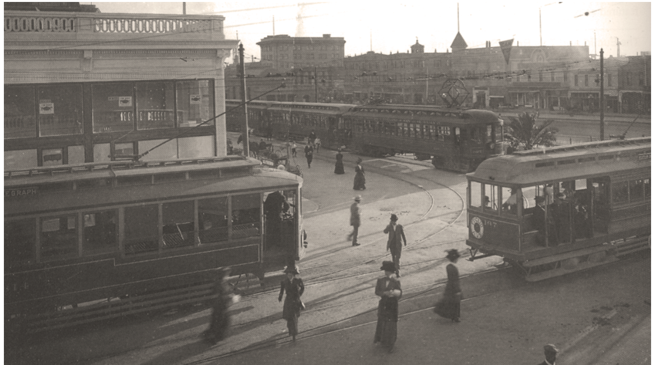
Figure HD-1: Berkeley Station Looking Southwest in 1910. Image courtesy of BAHA.
