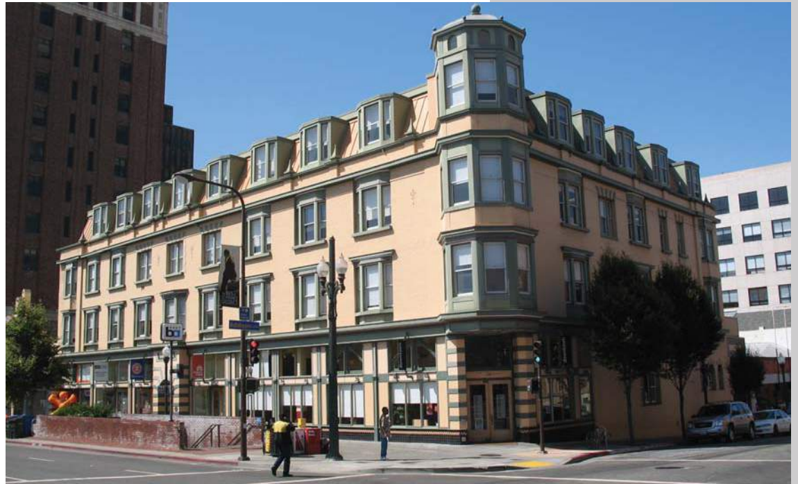
Figure HD-4: Adaptive Reuse & Intensification. The bottom three stories of the Francis K. Shattuck Building were built in 1901 and were renovated in 2000 at the same time as when a new fourth story was added. Staff photo
