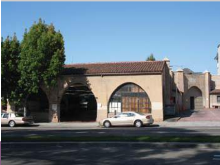
Figure LU-5: 1952 Oxford. University vehicles used to be maintained in this 1940 Mission Revival building designed by Walter Ratcliff. Staff photo.
