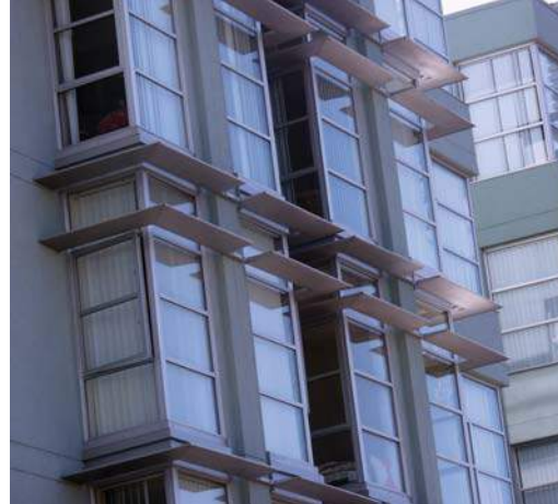
Figure HD-5: Historic Context & Green Features. The Fine Arts Building furthers a tradition of Art Deco buildings Downtown, and incorporates in a sympathetic way green features for energy efficiency, such as light shelves that bounce daylight deeply into interior spaces. Staff photos
